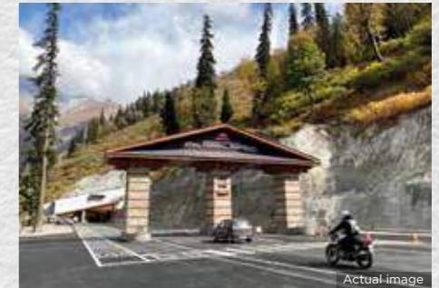
Atal Tunnel, Himachal Pradesh, 2020
