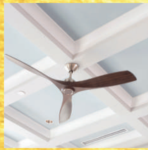
CEILING OIL BOUND DISTEMPER
