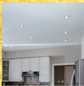
WALL / CEILING OIL BOUND DISTEMPER
